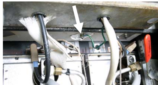
Figure 2: The burner ground on the module is grounded to the new ground stud and an existing fry pot stud (see arrow).
